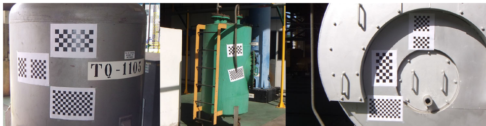
Fig. 18 Optical markers placed in simulated industrial environment at Petrobras' Research Center (CENPES). Left storage tank. Center pressure vessel. Right heat exchanger
