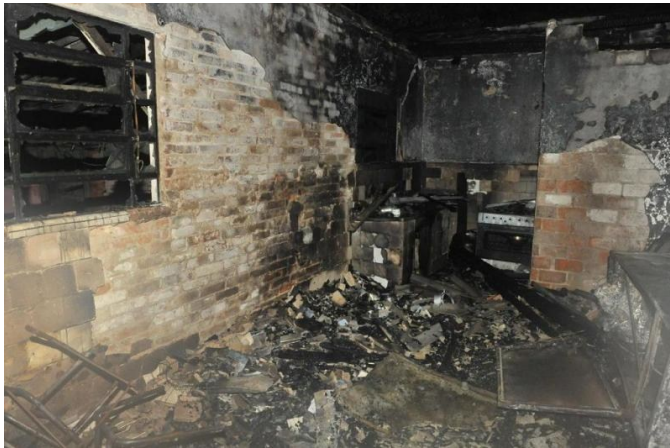
Fig. 8. Photo recorded by a local newspaper showing a house that caught fire after a short-circuit in the power network caused by lightning strike ( http://zerohora.clicrbs.com.br/rs/fotos/veja-fotos-do-mau-tempo-no-rs-durante-a-madrugada-34544.html ).
