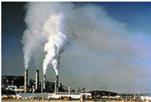
Figure 1: Before flue gas desulfurization was installed, the emissions from this power plant in New Mexico contained excessive amounts of Sulfur Dioxide. (Font: http://en.wikipedia.org/wiki/Air_pollution ).
