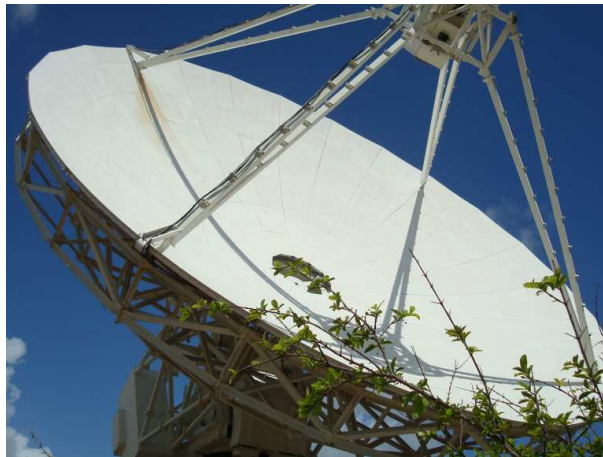
Figure 1. Fortaleza's 14.2 m antenna.
