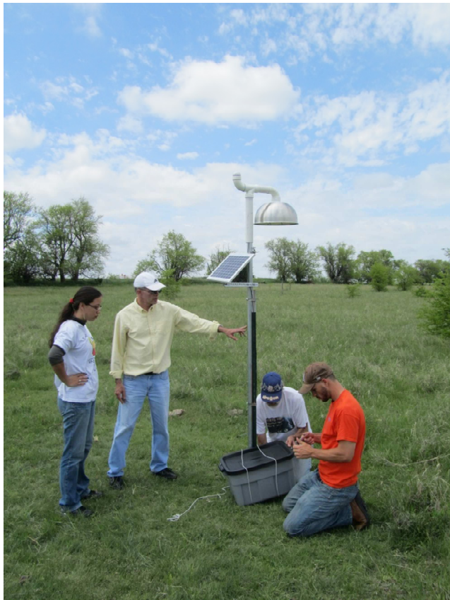
Fig. 6. New Mexico Tech solar-powered slow antenna installation. Battery box is being installed by Ron Thomas and Mason Quick, while being well-managed by our illustrious Brazilian team.
