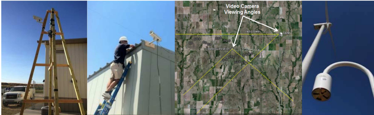
Fig. 2. (From Left to Right) Video camera installation at the Operations & Maintenance Building; video camera installation at the sub-station; map of the video camera viewing angles; view of an electric field mill installed at the wind farm
